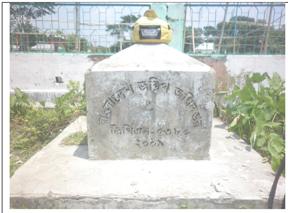
Plate-2: Reference BM Pillar (GPS-5380) of SoB in Ishwarganj Upazila
