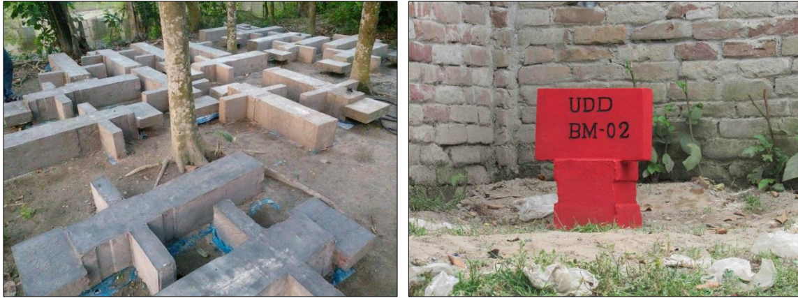
Plate 1: Sample of Constructed BM and Installed BM
