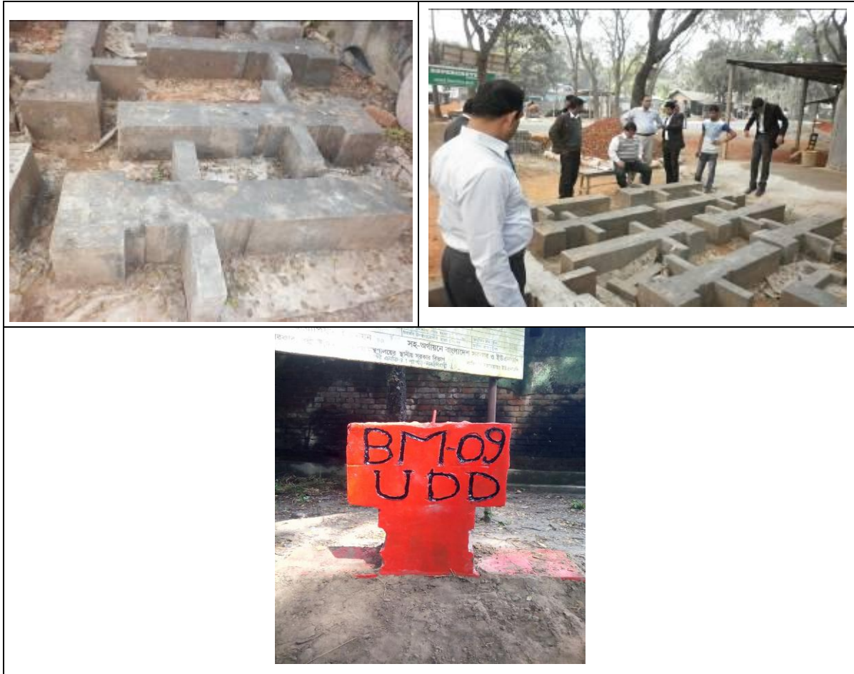
Plate-1: Sample of Constructed BM and Installed BM
